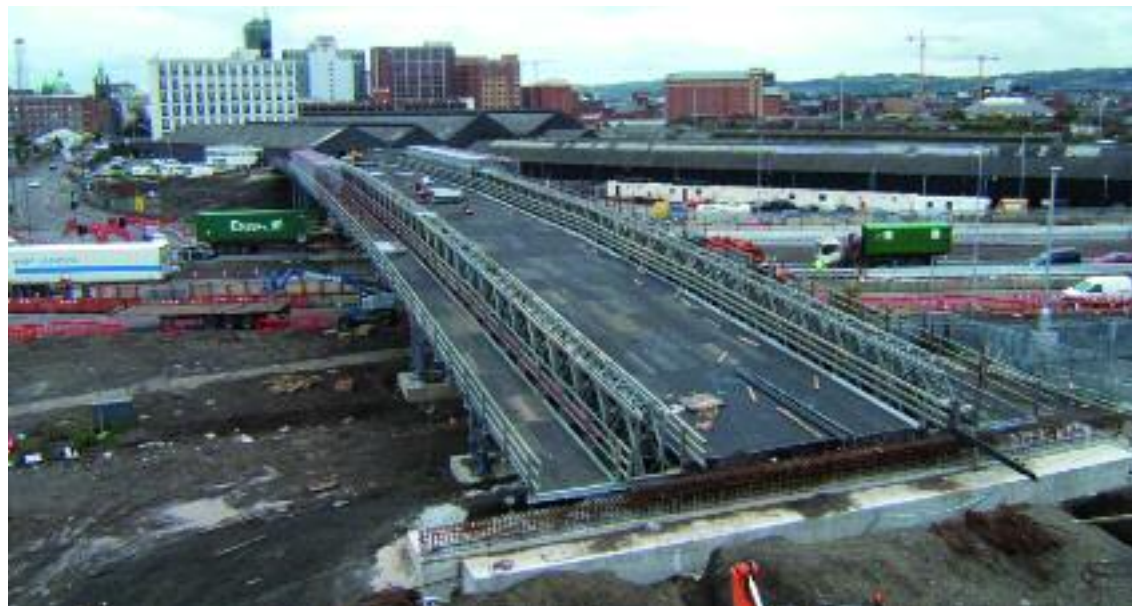
The new temporary Bailey bridge at Grosvenor Road just prior to opening
